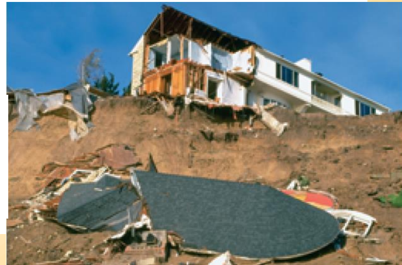
Figure 19 Landslide This home in Pacific Palisades, California, was destroyed by a landslide triggered by the January 1994 Northridge earthquake.
