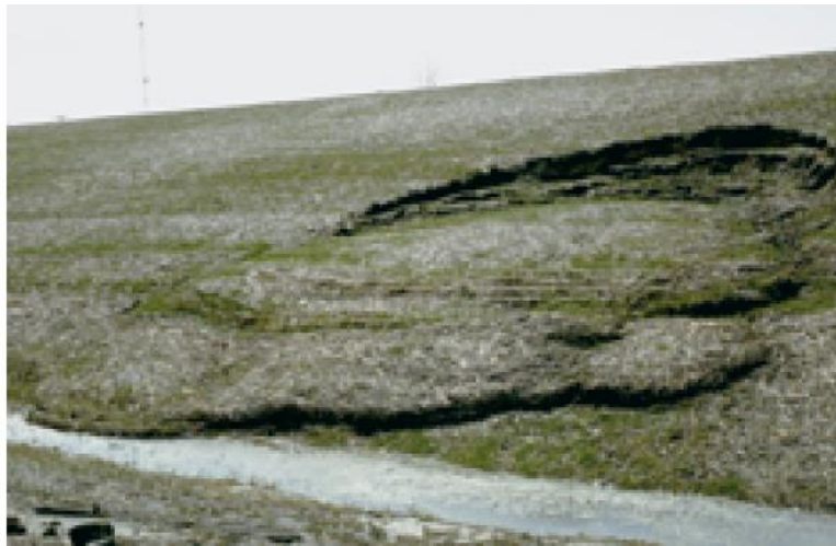
Figure 23 Earthflow This small, tongue-shaped mass movement occurred on a newly formed slope along a recently built highway.
